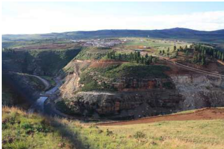
Metolong Dam under construction
