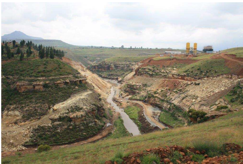
Metolong Dam under construction
