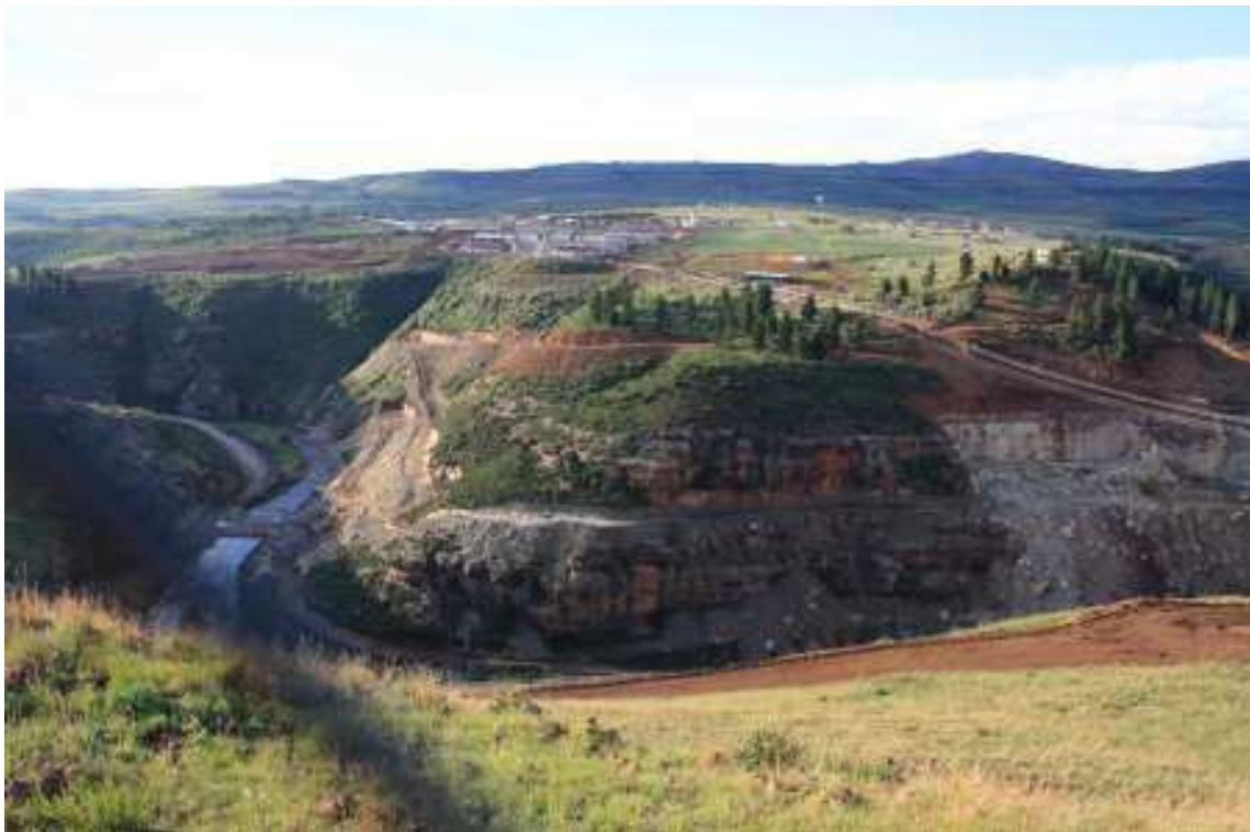
Metolong Dam under construction
