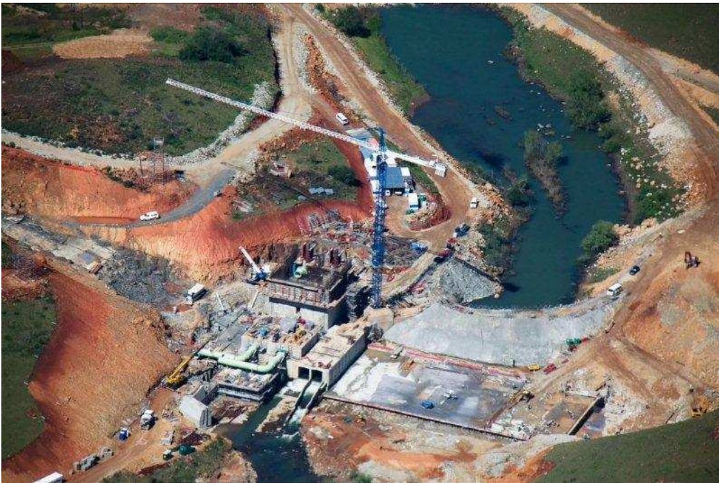
Spring Grove Dam under construction
