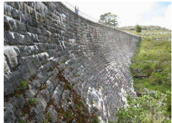
Downstream face of Hely-Hutchinson Dam
