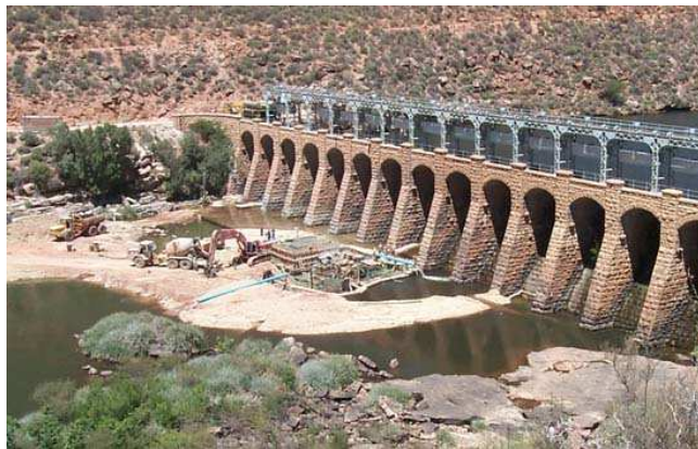
Remedial work at the Bulshoek Dam 2004
